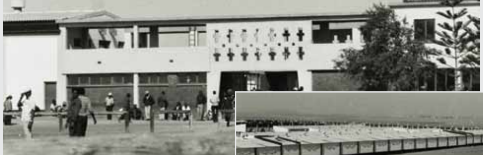
The façade of workers compound 1970's with contract workers in the foreground
