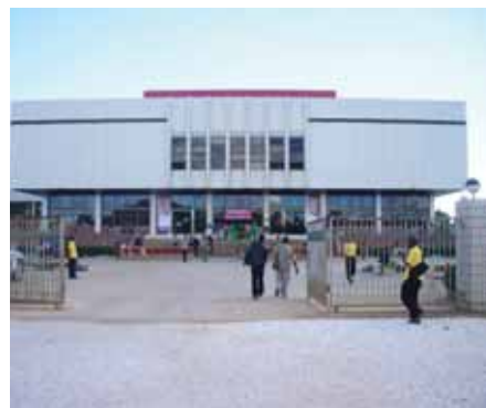
Lusaka National Museum Building
