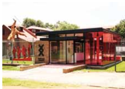
The outside of the Workers Museum with its new Visitors' Centre. Copyright: Workers Museum
